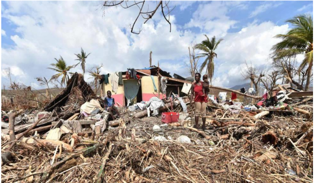
Aftermath passage major Hurricane Matthew 2016 over southwestern Haiti
