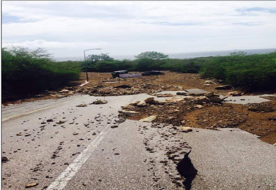
*Picture of a road washed away in Bandabou, due to flash flood on November 28, 2015
