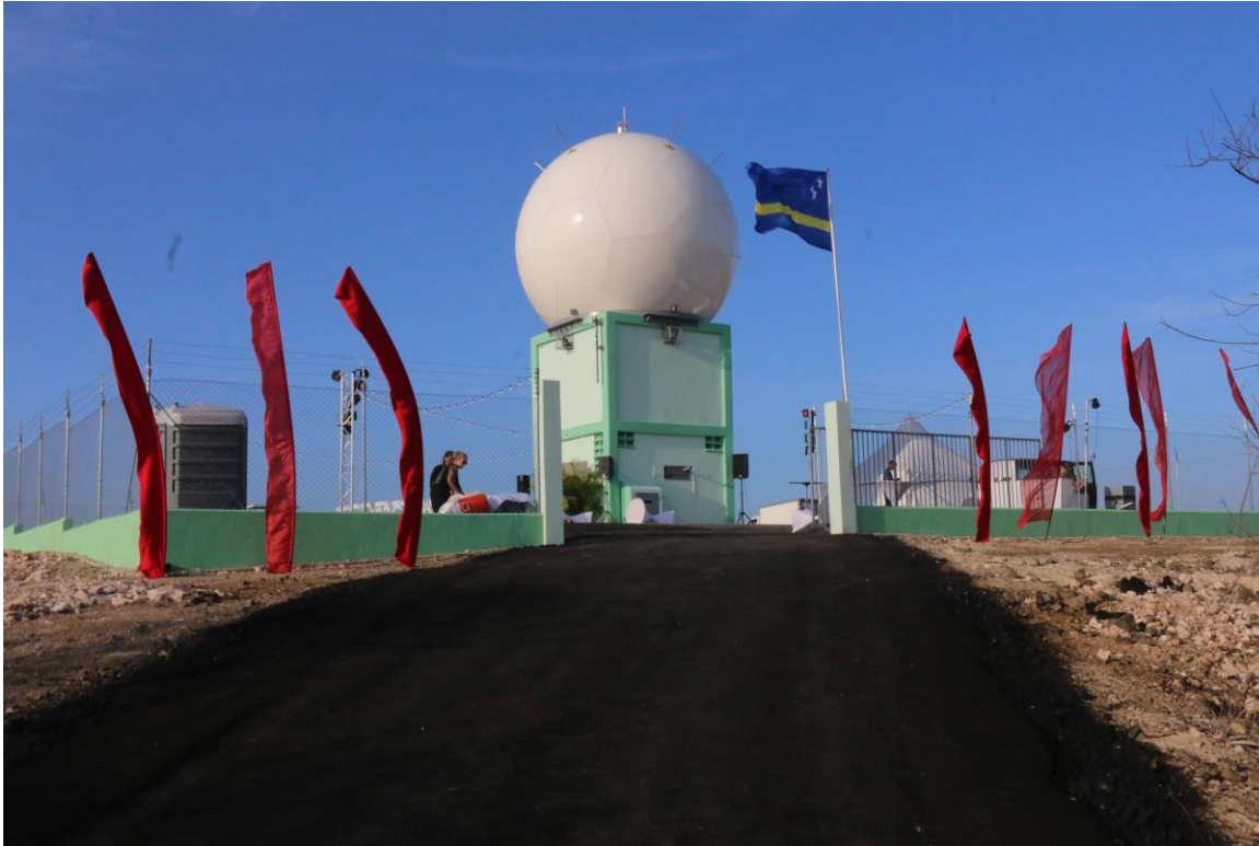
The renovated radar site on Seru Spelonk, near the Hato caves
