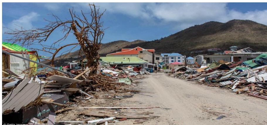
Completely levelled neighborhood, St. Maarten, Hurricane IRMA 2017
